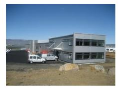
Contract between JÁVERK ehf. and the Client in General Contract. Concrete work and finish work inside and outside for completion. The structural load-bearing construction is of steel. Facades claddings of rockwool sandwich-elements. The project was handed out to the client in february 2007. Total area: 4.160m2. Client: Íslensk Ameríska hf <u>www.isam.is</u> Client's supervision: Hjalti Nielsen, CEO.
