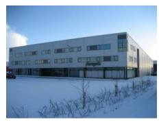
Tender in General Contract. Concrete work on foundations and stairways. Lc bearing construction in outer walls and roof of steel. Outer walls cladded by sandwich-elements and aluminum sheets. All windows of aluminum profiles The project was handed out to the client in april 2008. Total area: 4.299m2. Client: Uppruni ehf. www.europris.is Client's supervision: Júlíus Bernburg, Conís Consulting engineers.
