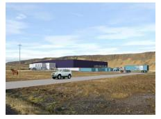
Tender in Turnkey Contract. Design of the project in co-operation with Architect company Tröð in Reykjavik. Earth and concrete works and finish work of the construction inside and outside. The structural load-bearing construction is of combined concrete-elements and steel. Roof structural construction is of truss girders of steel.
