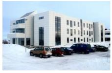
Tender in General Contract. Extension to the hospital in Selfoss. The loadbearing construction is of concrete. Finish work outside and inside. The project was handed out to the client in february 2007. Total area: 5.469m2.
