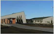
Tender in General Contract. Concrete work and finish work inside and outside for completion and the structure connected to existing building. Load bearing structure of concrete and gluelam beams. The project was handed out to the client in juli 2005. Total area: 1.408m2. Client: Rangárþing Eystra <u>www.hvolsvollur.is</u> Client's supervision: Rúnar Guðmundsson, Hvolsvöllur County hall.
