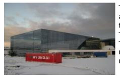
Tender in General Contract. Earth- and concrete work, finish work inside and outside for completion. The load bearing construction of steel and the facades cladded with glass construction. The project was handed out to the client in September 2008. Total area: 7.000m2. Client: Borgarhöllin ehf. Client's supervision: Erlendur Fjeldsted.
