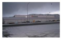
Contract between JÁVERK ehf. and the Client in General Contract. Concrete work of foundations and finish work for completion inside and outside. Load bearing structure of walls and roof construction is of gluelam. Claddings in outer walls of sandwich-elements and roof insulated and cladded with steel sheets. The project was handed out to the client in may 2001. Total area: 3.500m2. Client: Húsasmiðjan hf <u>www.husa.is</u> Client's supervision: Steinar Árnason, Húsasmiðjan hf.
